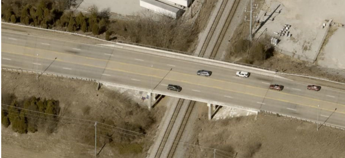
Figure 13: US 231 over CSX Rail lines
