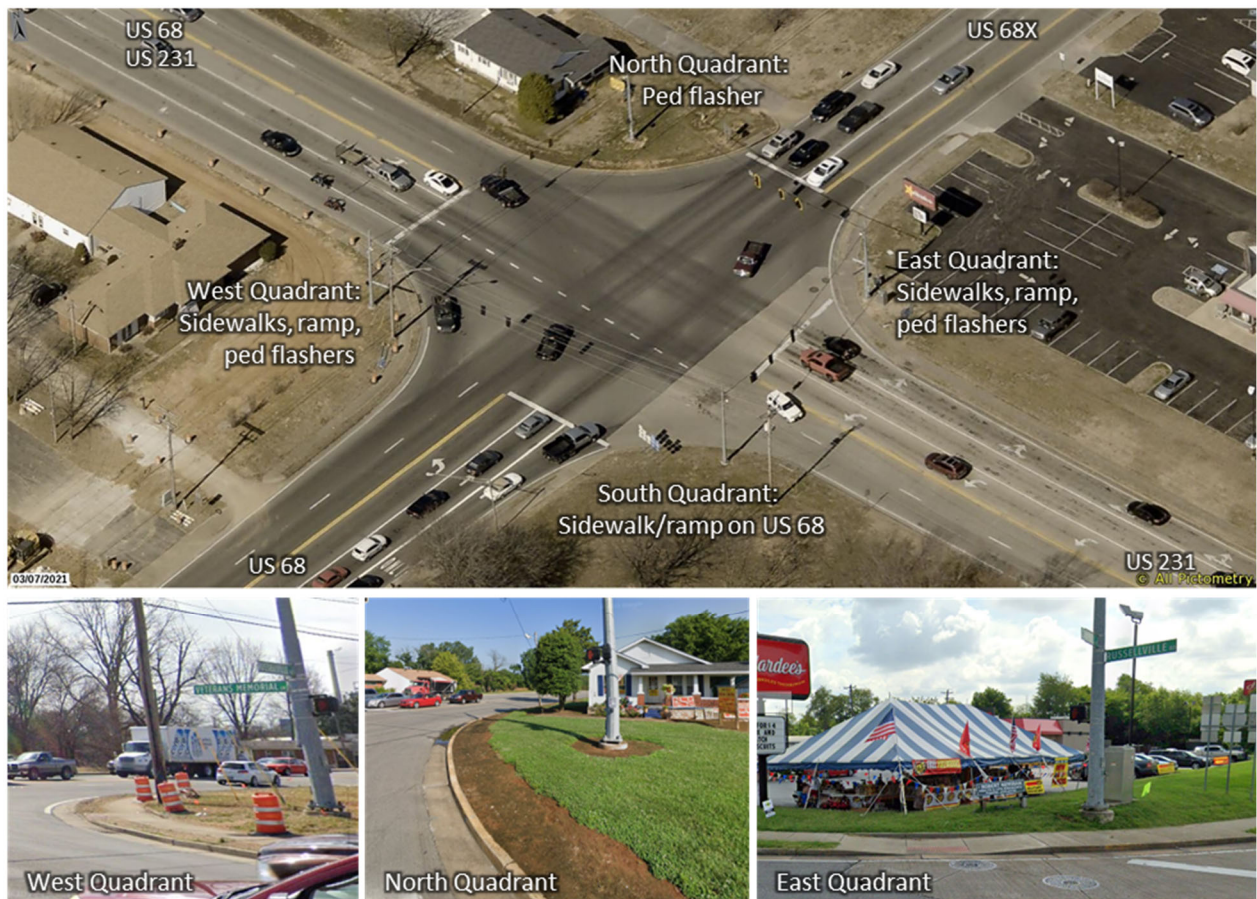
Figure 6: Existing Pedestrian Facilities
